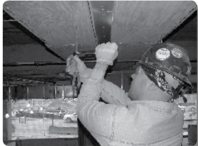
Problem: Tightening conventional nut on all-thread
