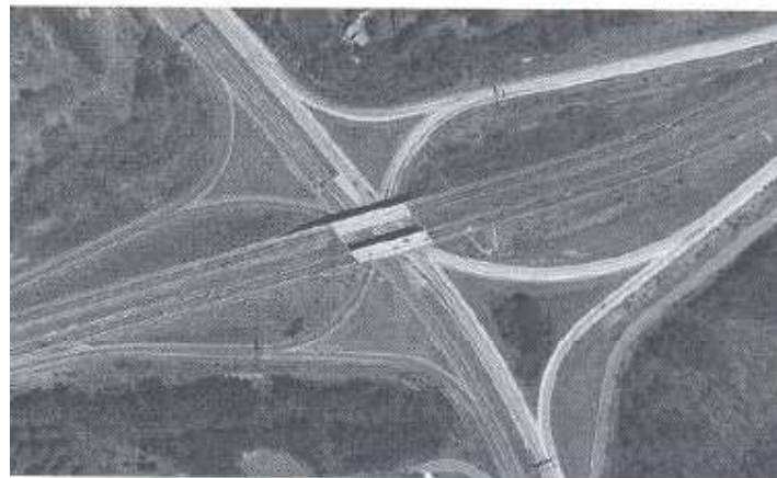
– B – Overpass SPDI
